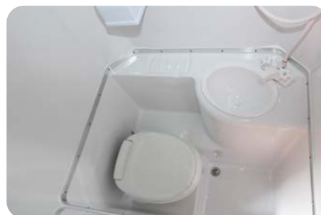
Bathroom with Sink, Toilet, and Shower
