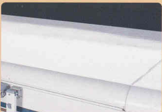
1-year old Itasca fiberglass roof
