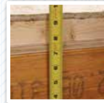
7" HEADER BEAM VS. 2" X 6" LUMBER
