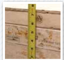
7" HEADER BEAM VS. 2" X 6" LUMBER
