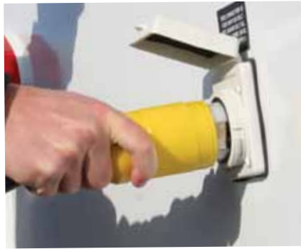
50 AMP service, ready for second air conditioner
